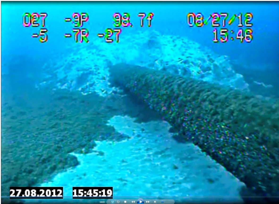
Figure 30. Frame Grab from Enbridge 2012 Underwater Inspection Video 24 of the East Leg of Line 5 under the Straits of Mackinac Depicting a Clay Pile
