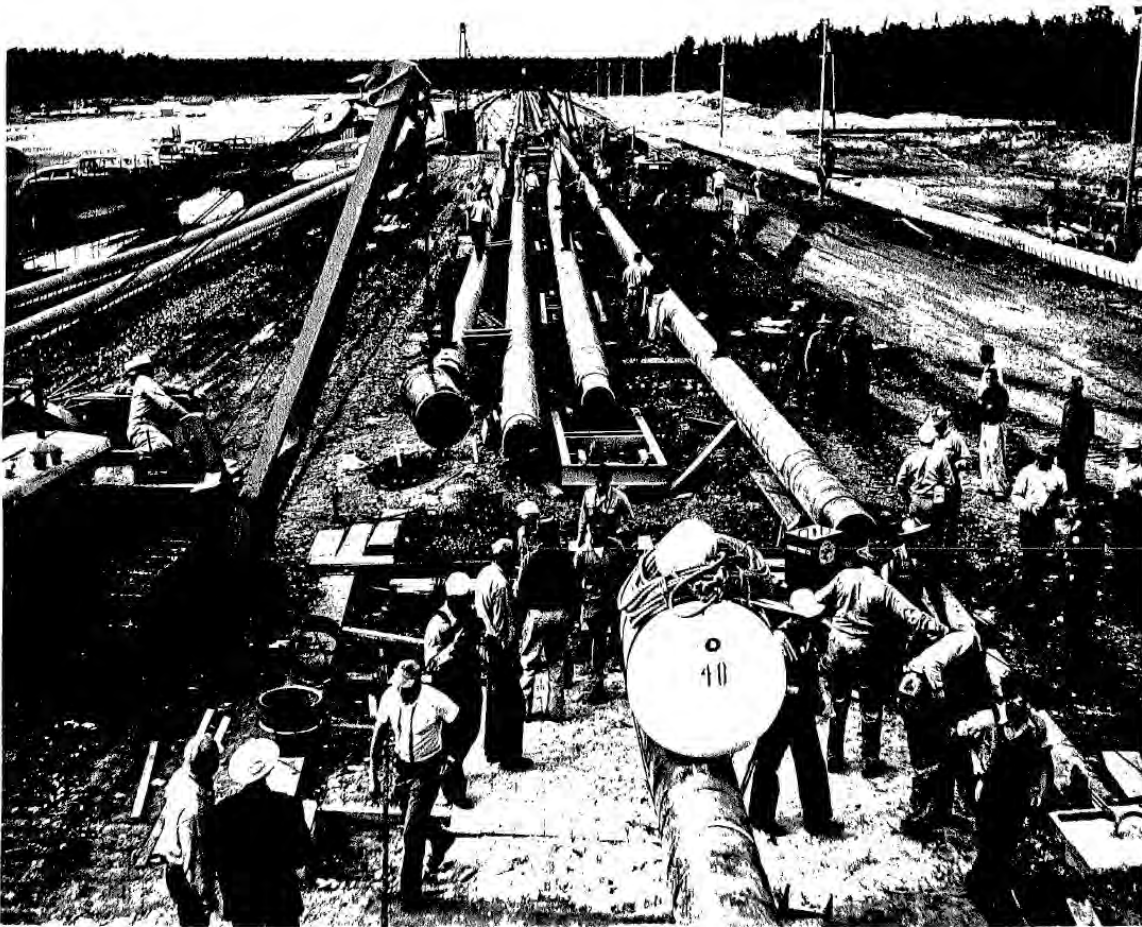
Figure 29. 1953 Photograph Showing Curvature of Pipe String as it is Moved onto the Launch Way Using a Crane
