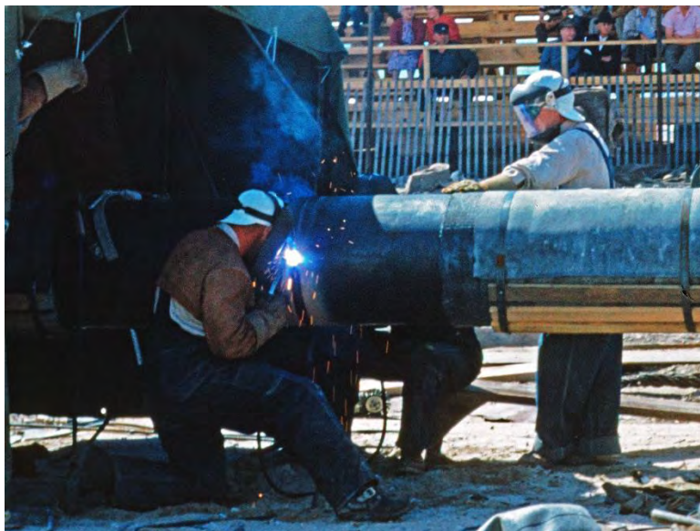
Figure 5. Trudgen Photo of Pipe String Assembly Welding (00010370005.tif)
