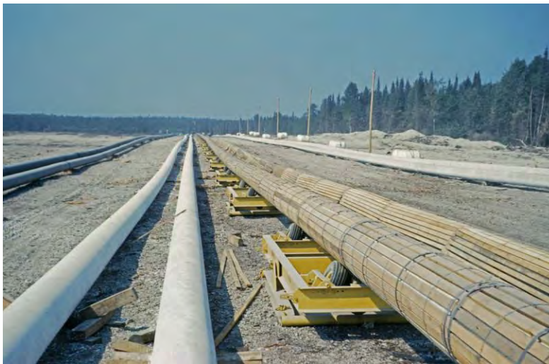
Figure 4. Trudgen Photo of Pipe Stockyard (00010370011.tif)
