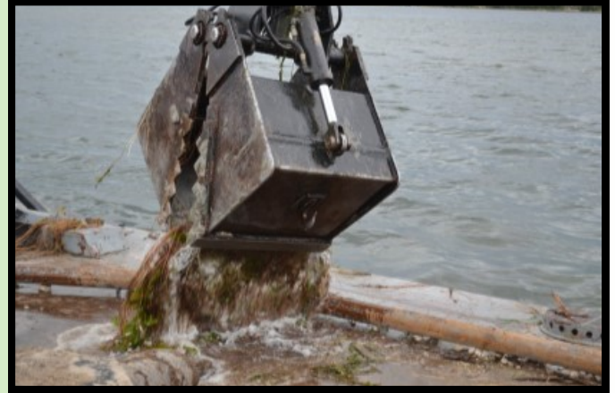
Dredging EWM in Federal Navigation Channel
